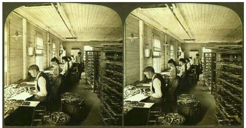
A corner of the finish and varnishing room for making stereoscopes
